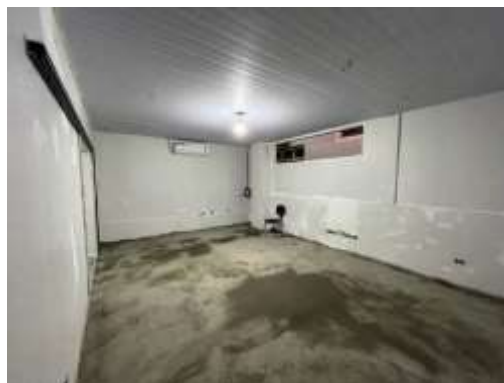
Reforma GAPS e GECEV
